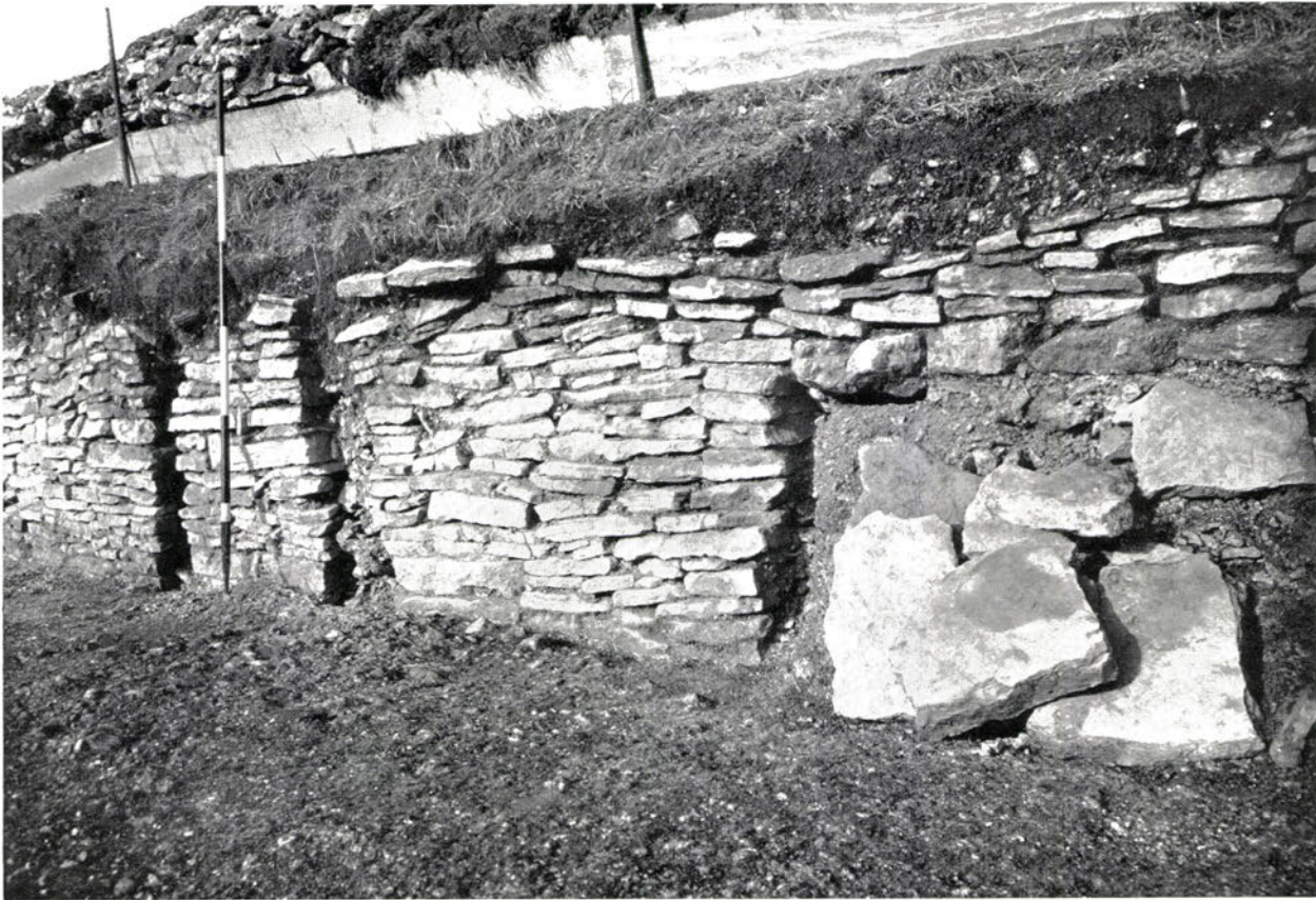
A. Eastern entrance: Iron Age A walling on the outer face of the hornwork, showing the sockets for posts and (on the right) a rebuilding after the decay of a post and the collapse of the wall. See pp. 38, 110
