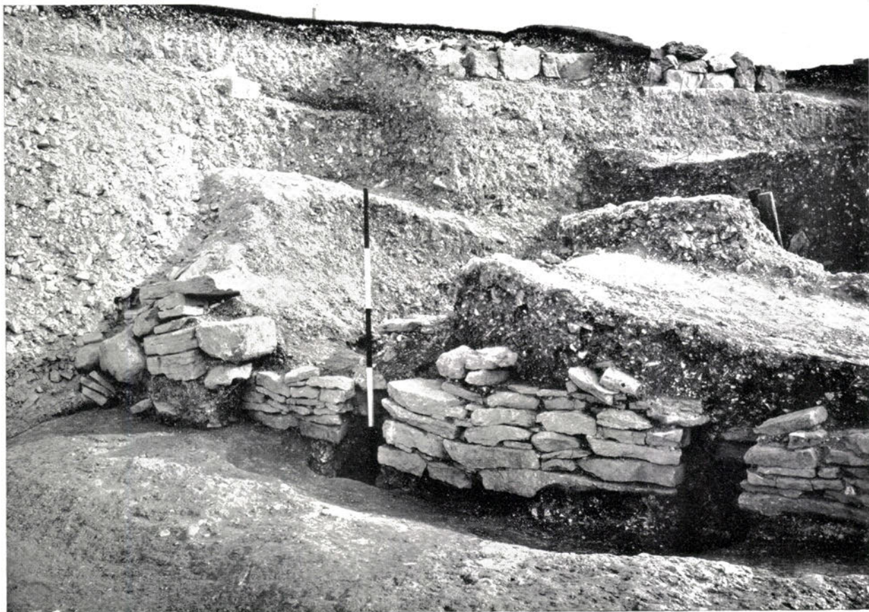
Eastern entrance: flank of the Iron Age A road through the hornwork, showing post-holes and walling of Iron Age A and (on left) Iron Age B repairs to walling. See pp. 45, 110
