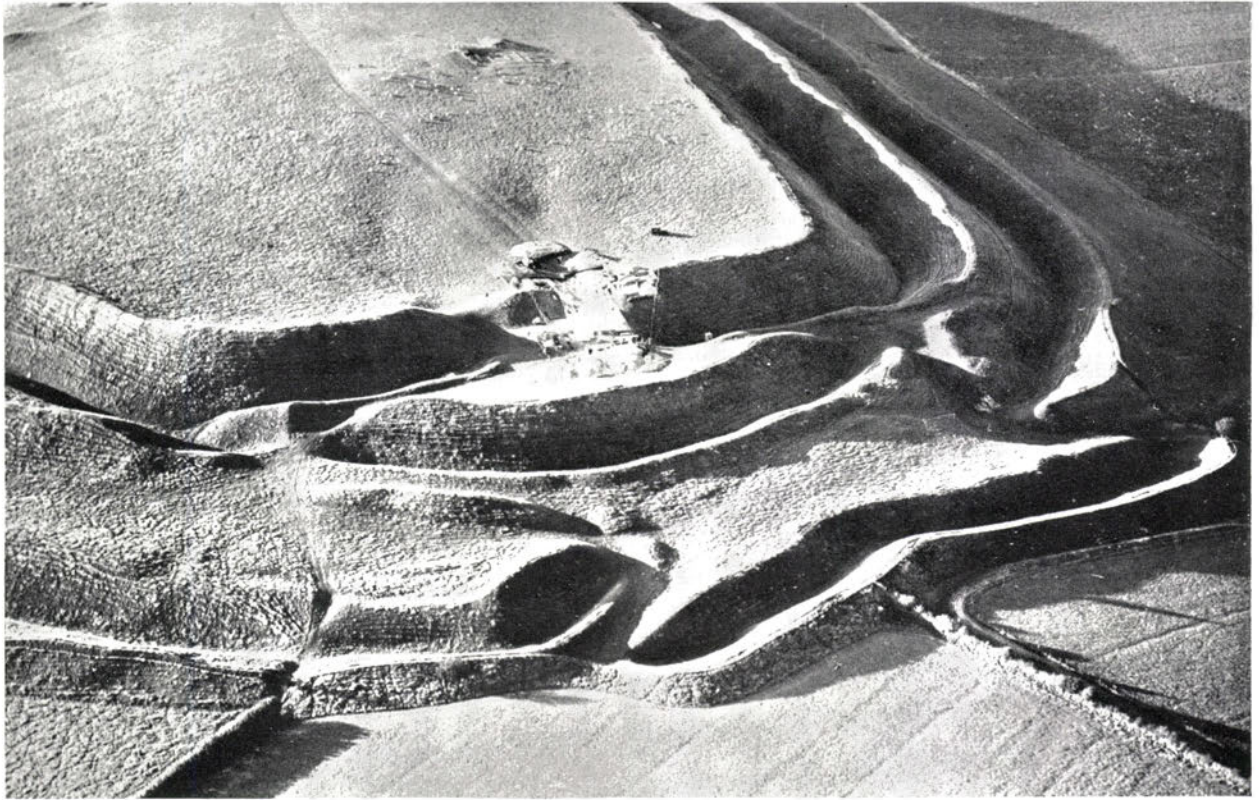
A. Eastern entrance from the S.E., during excavation
